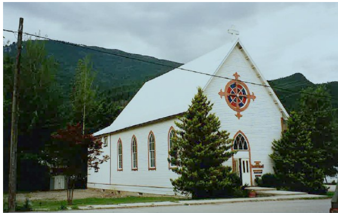
Sacred Heart Mission, Kaslo B.C. (originally built in 1893, this Church replaced it in 1902, Photo 1990s, Diocese of Nelson, B.C. Archives
